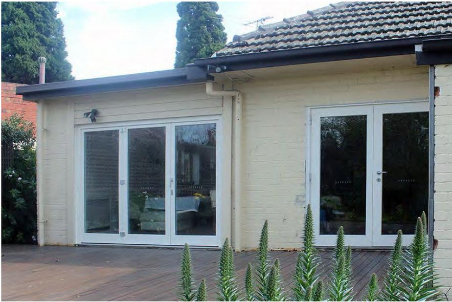
Rebated frames, seals, multi-point locking and double or triple glazing ensure the highest energy efficiency with no rattling. Operated with a handle on every second door, there is no need for shoot bolts.
